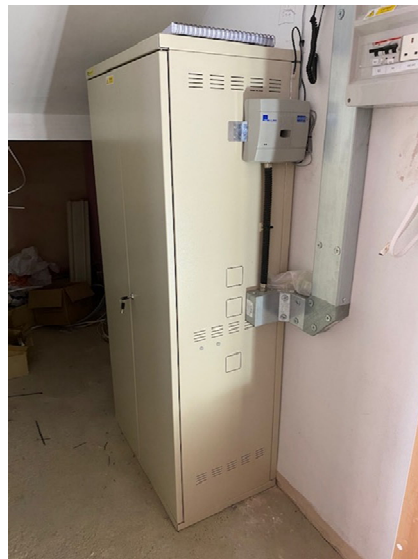
MINI USED FOR MACHINE ROOM CABINET AND HOME LIFT APPLICATIONS
