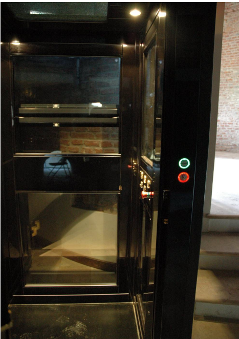
Panoramic cabin, black mirror stainless steel finishings, LED spots horizontal station panel
